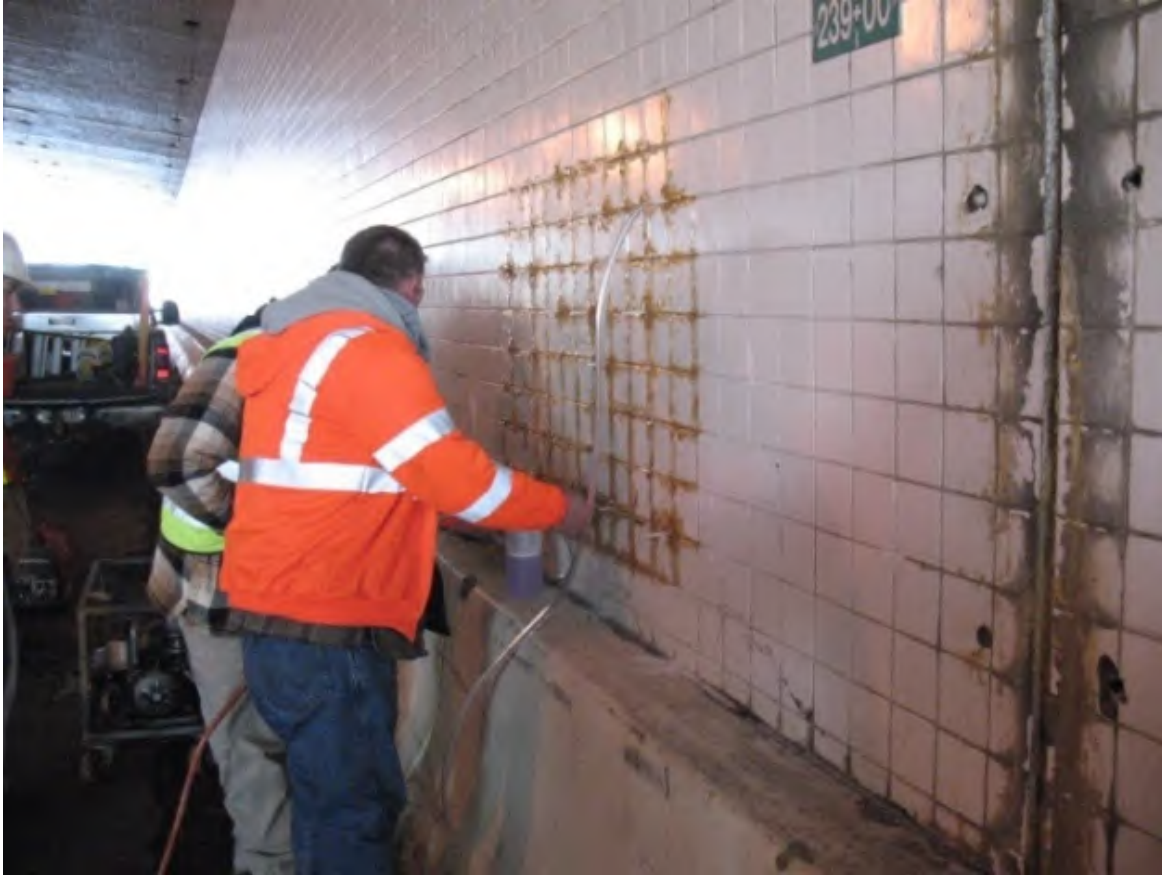
Figure 3.27 – Vacuum Injection with Methyl Methacrylate (NCHRP, 2010).
