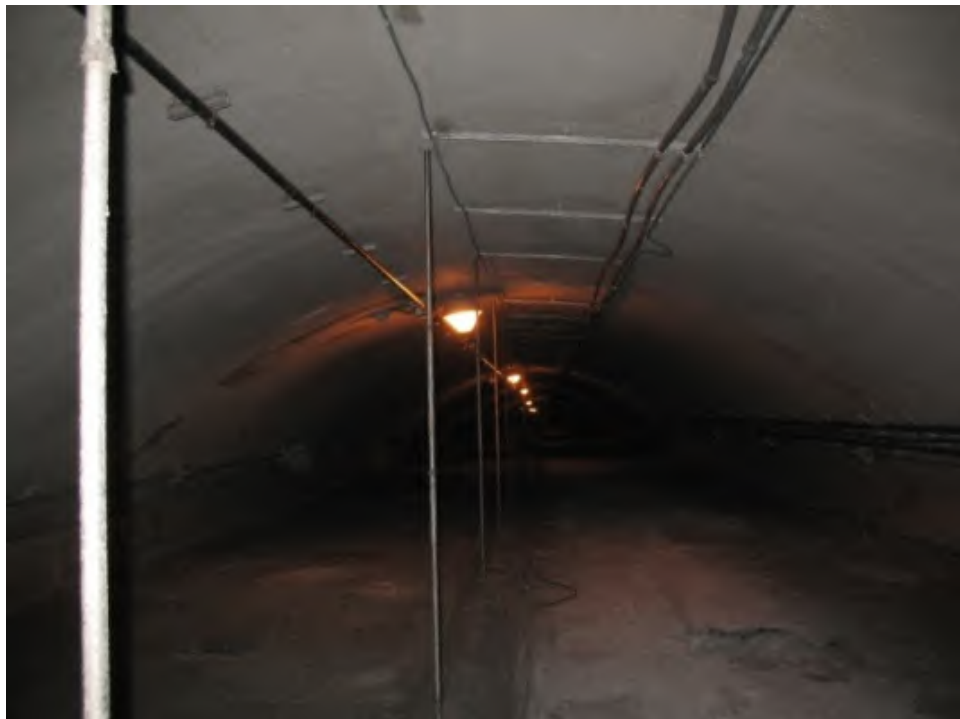
Figure 3.23 –View of a cementitious coating applied to the arch (NCHRP, 2010).
