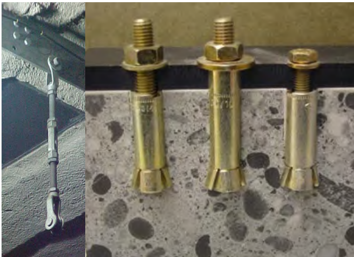
Figure 3.30 – Typical replacement hardware left; undercut mechanical anchors, right.
