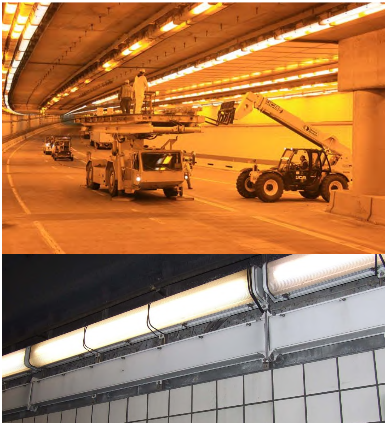
Figure 3.33 – Tunnel lighting maintenance and cleaning.
